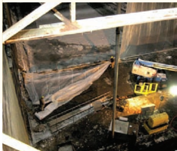
Winter work begins at the locks with the crew hanging plastic curtains to isolate the work area.
