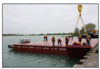
Corporation personnel under the direction of Poseidon representatives are assembling the sectional spud barge for the first time.
