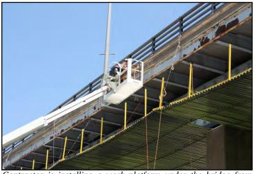
Contractor is installing a work platform under the bridge from which to perform blast cleaning and painting operations.
