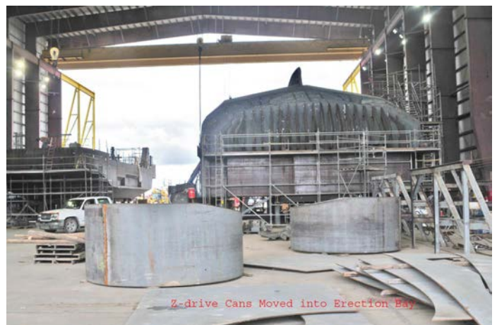
Stern view with Z-Drive cans being prepared for installation.
