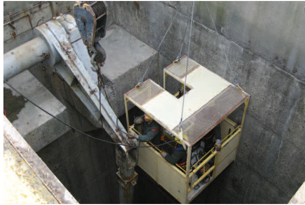
Preparing to remove the valve stem for repair.
