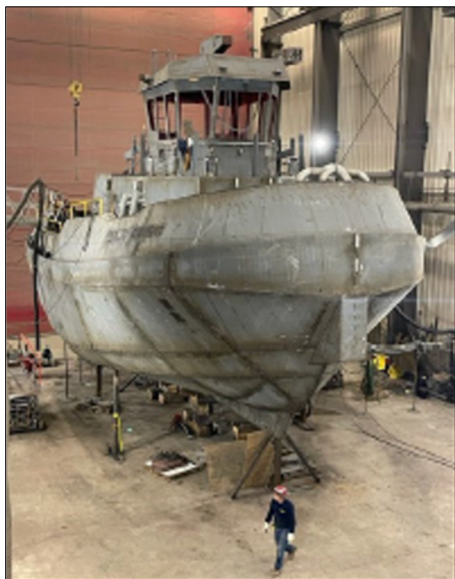
The GLS’s new 60-foot tugboat, Seaway Guardian, under construction at the Washburn & Doughty Associates shipyard in East Boothbay, Maine.
