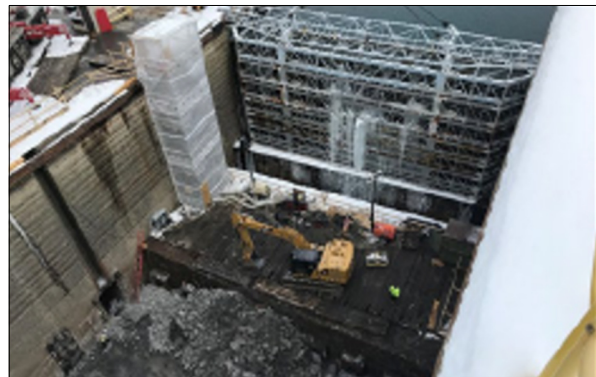
Work crews performing the rehabilitation of the diffusers at Eisenhower Lock.
