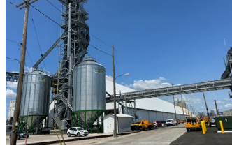
Port Milwaukee, FY19 PIDP-funded project completed.
