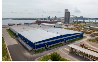
Duluth Seaway Port Authority, FY19 PIDP-funded building project completed.
