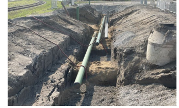
Toledo-Lucas County Port Authority, FY19 PIDP-funded project in progress.
