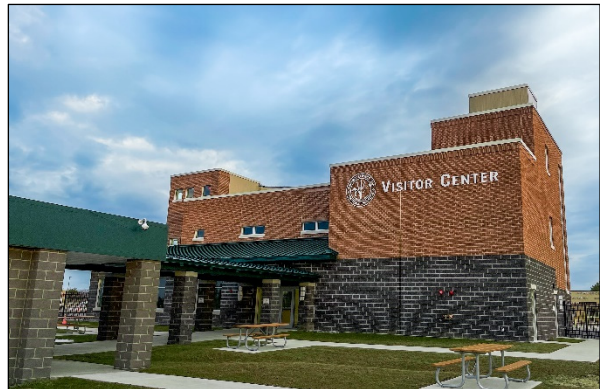
The GLS's Seaway Visitor Center at Eisenhower Lock was completed in early FY 2024 and opened to the public in May 2024.
